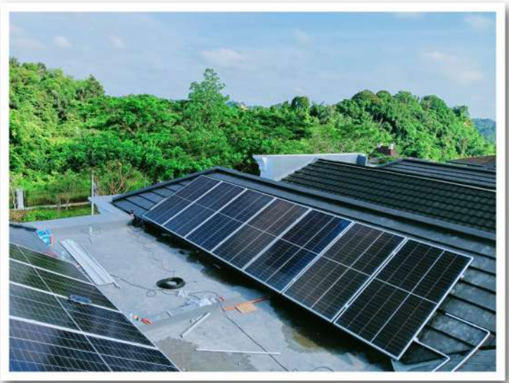
@ Samarinda - 10 kW On Grid 3 phase
